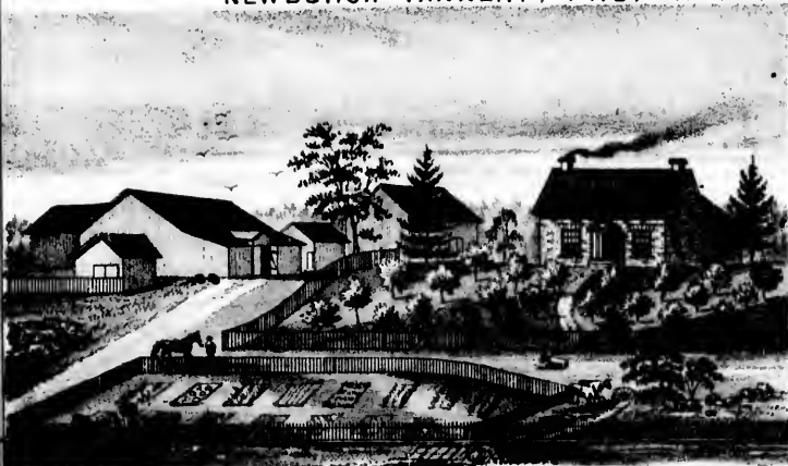
FARM RESIDENCE OF A. SPIKE, PORTLAND TW'P. ONT.
